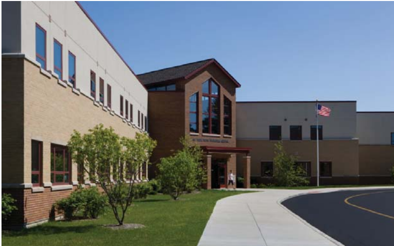
Building addition to St. Bede Faith Formation Center Ingleside, Illinois
